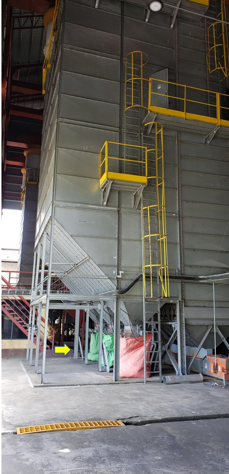
<Figure 44: Dust Accumulation Systems at Base of Tower Dryer>
