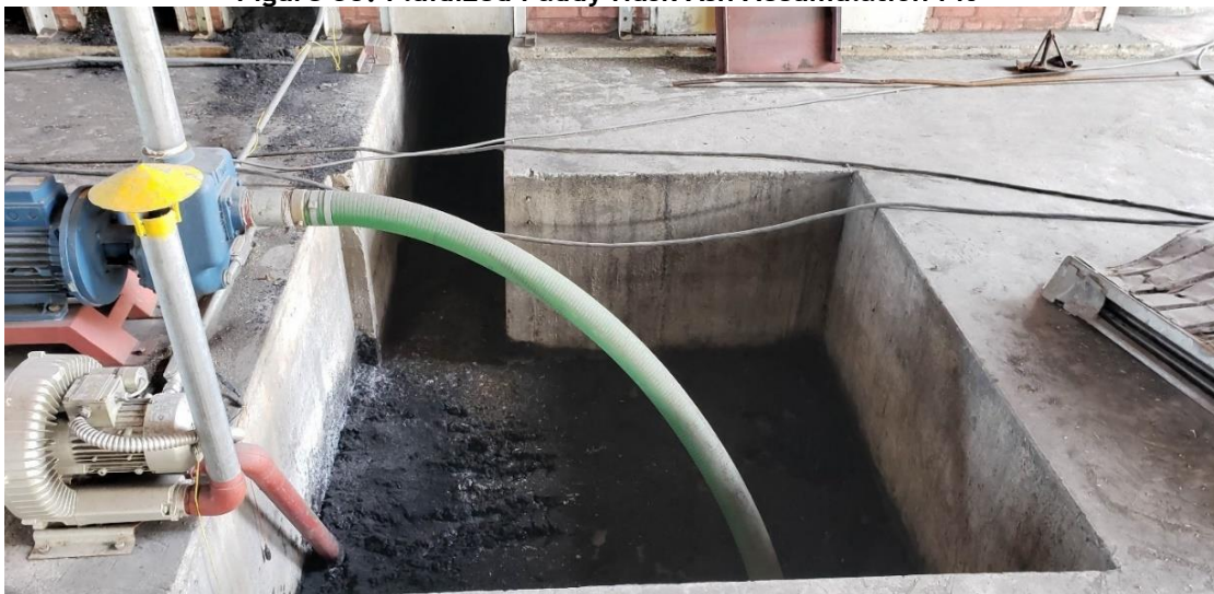
Figure 33: Fluidized Paddy Husk Ash Accumulation Pit>
