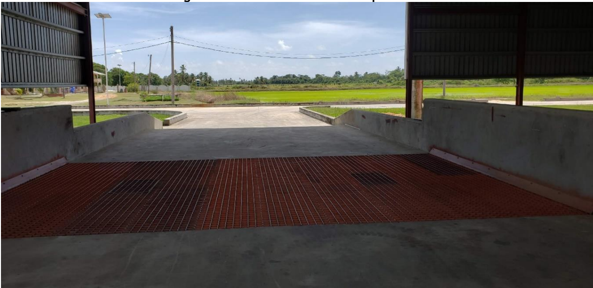
<Figure 8: Grates over Grain Reception Pit>
