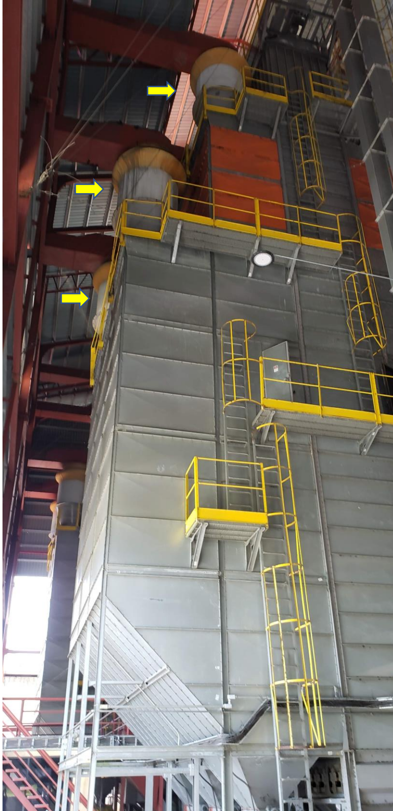
<Figure 43: Vortex Collection System atop Tower Dryer for Dust Capture>
