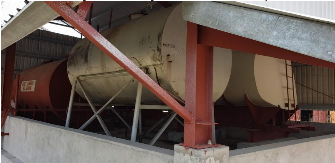
<Figure 38: Aboveground Fuel Storage Tanks in Covered Secondary Containment>
