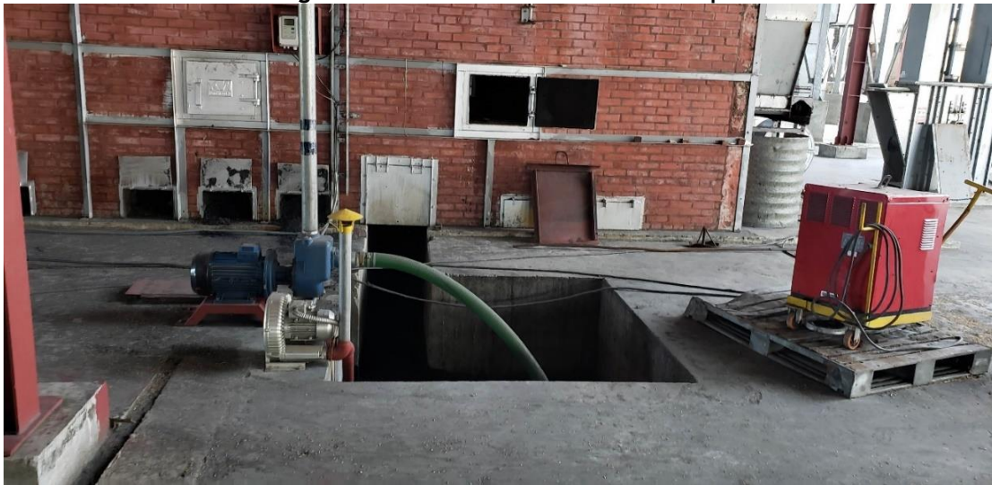
<Figure 32: Air Blower and Suction Pump>
